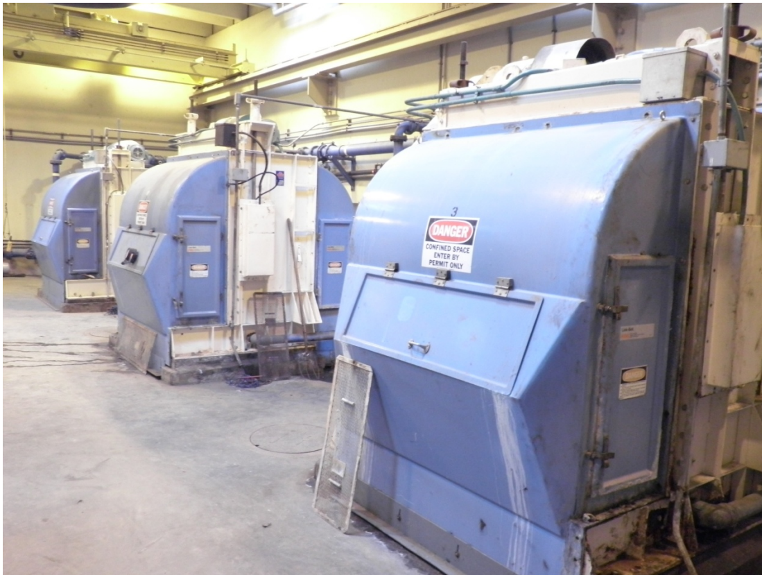
Photo 3.3 Three travelling screens located inside the low service building
