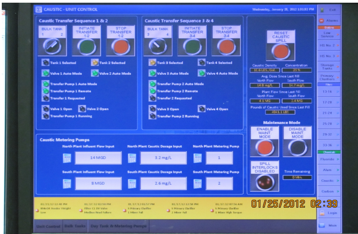
Operator's Control Room
