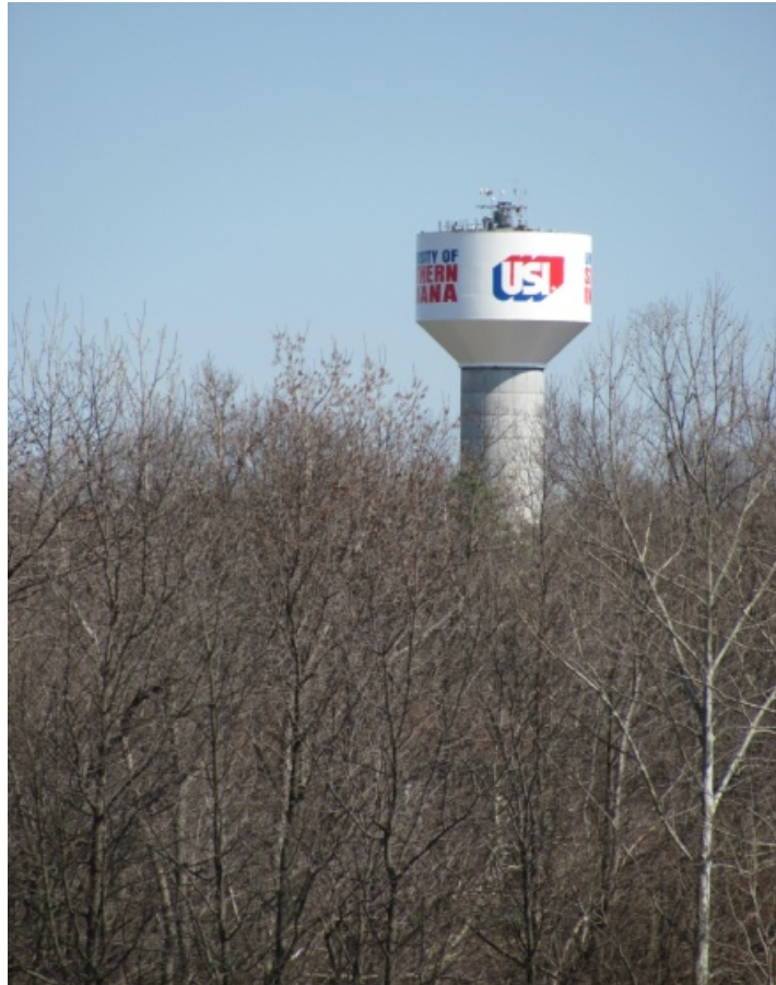
Photo 11.4 USI Tank - 0.5 Million Gallon Water Tower
