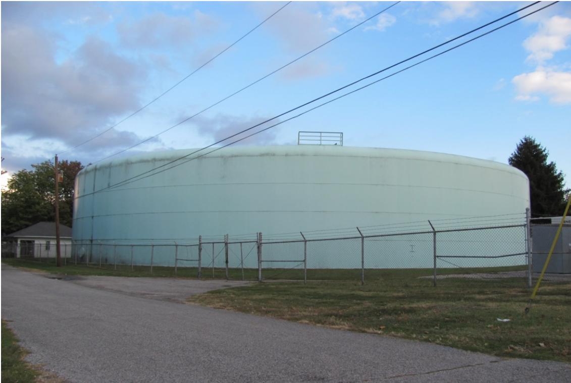
Photo 11.2 Killian Reservoir – 4 Million Gallon above Ground Reservoir
