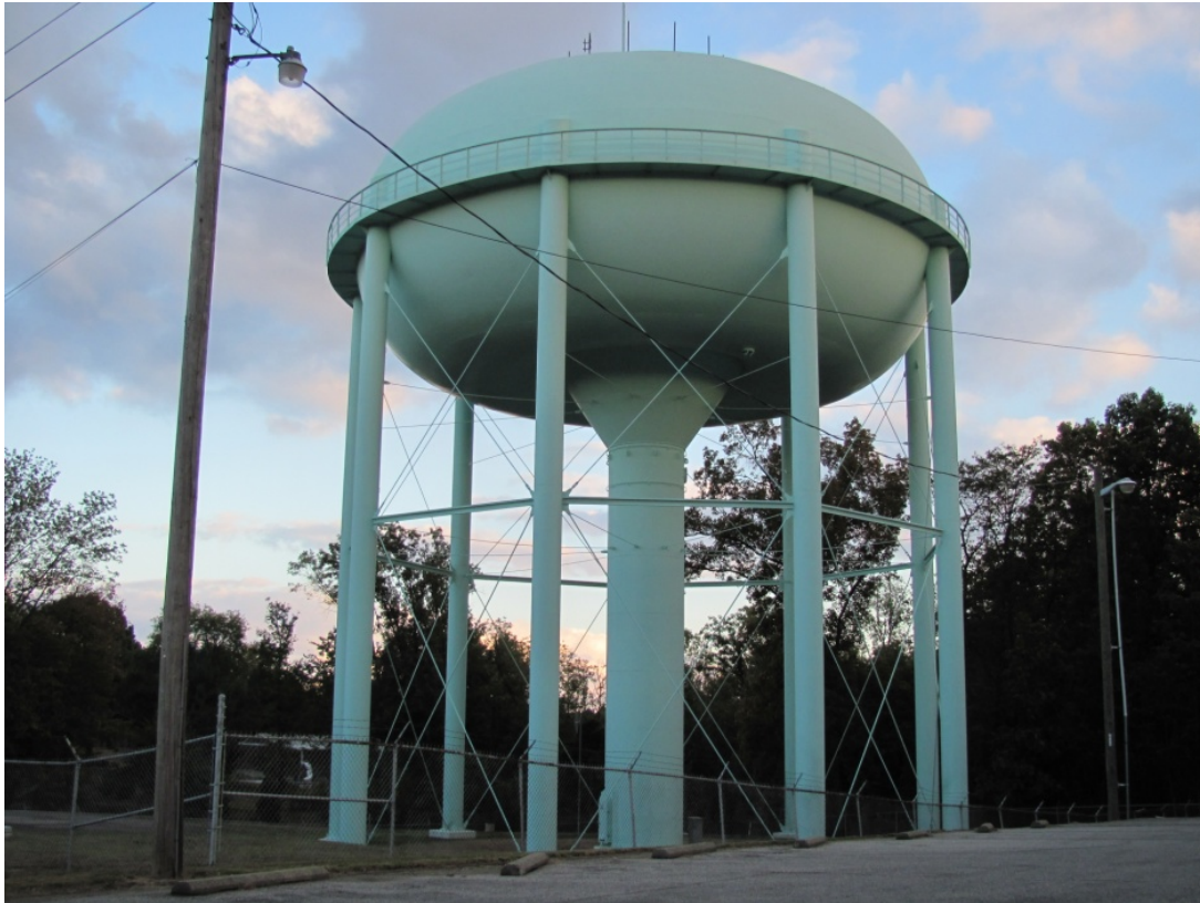
Photo 11.1 Darmstadt Tank - 1.0 Million Gallon Water Tower
