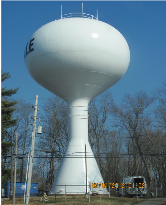
Photo 11.6 Upper Mt. Vernon Tank - 0.5 Million Gallon Water Tower
