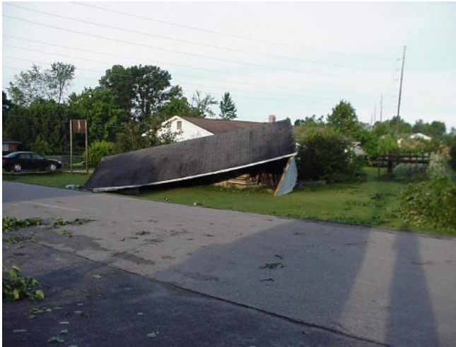
Figure 3.28 Roof Blown Off A House Located In the City of Darmstadt, May 30, 2004
