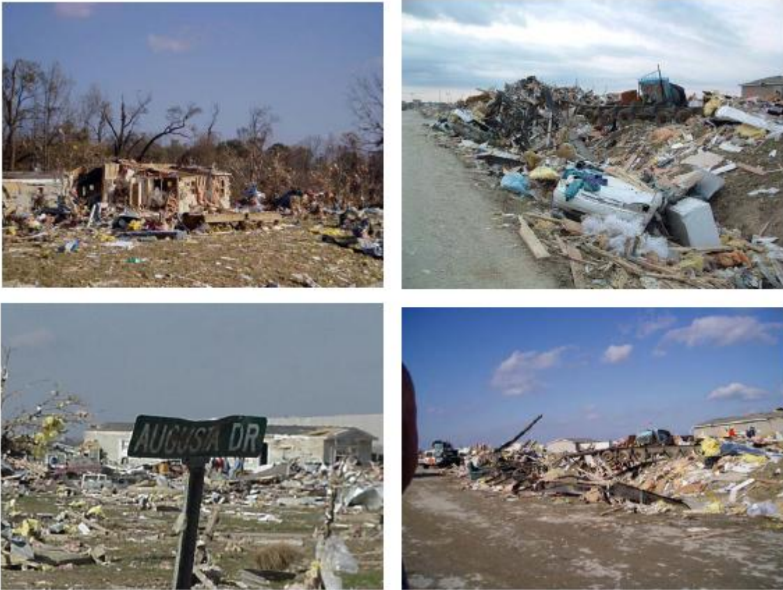
Figure 3.27 Tornado Damage at the Eastbrooke Mobile Home Park, November 6, 2006
