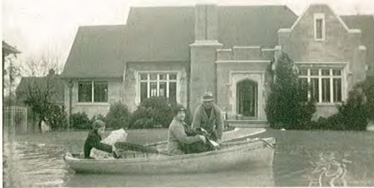
A street scene in front of the Albert Caden house at 631 Willow Road, during the great flood of 1937. (Photograph courtesy of Fred and Cathy Folz.)
