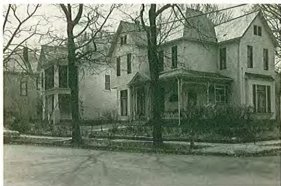
Built: 1891 Architecture: Queen Anne
