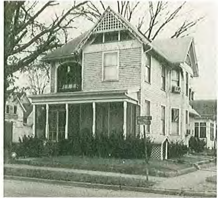
Built: 1890 Architecture: Queen Anne
