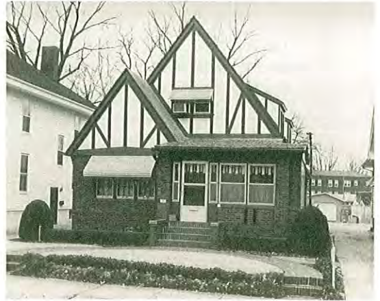
Built: 1927 Architecture: Tudor Revival
