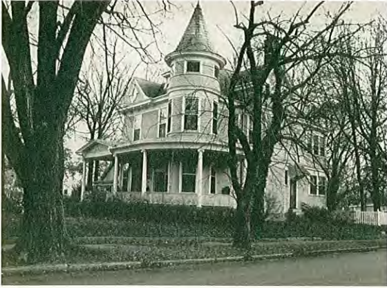
Built: 1902 Architecture: Queen Anne
