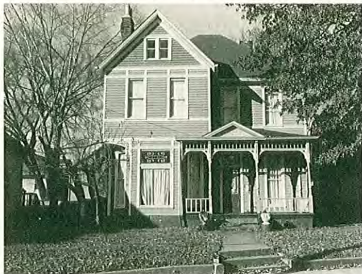
Built: 1892 Architecture: Queen Anne
