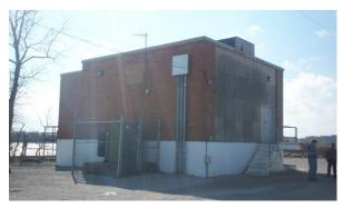
Another major project included in the plan is the replacement of the 7th Avenue Lift Station. This lift station, located south of the greenway trailhead near the mouth of Pigeon Creek, was constructed in 1955 and is one of the most critical pieces of sewer infrastructure in the Utility's system. The lift station has no onsite backup power system, and it has a single screen, with no redundancy, so it does not meet current
