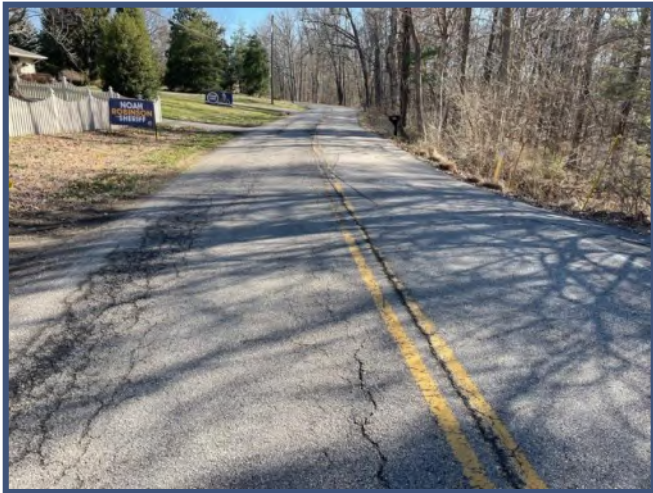
Near 3500 Koring Road
