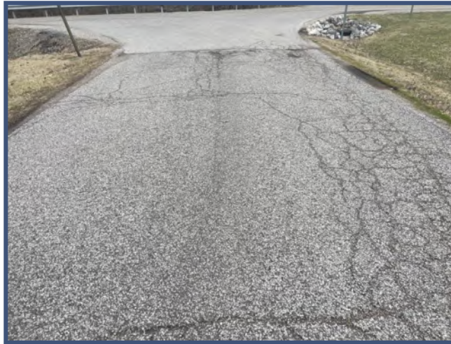
At S.R. 65 Intersection
