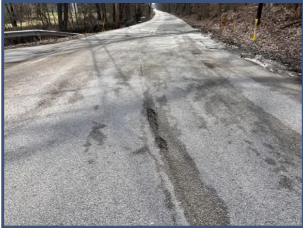
At Boehne Camp Road Intersection
